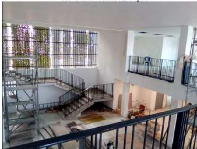
Vista de Interior- Hall Principal
