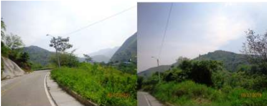
LUMINARIAS LED - VEREDA ANGELINOS
