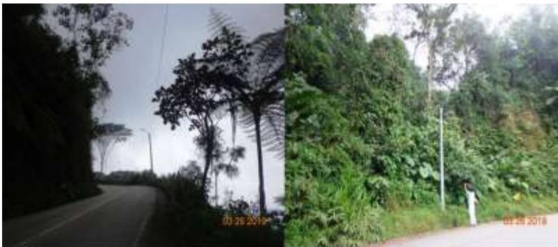
LUMINARIAS LED - VEREDA RETIRO GRANDE
